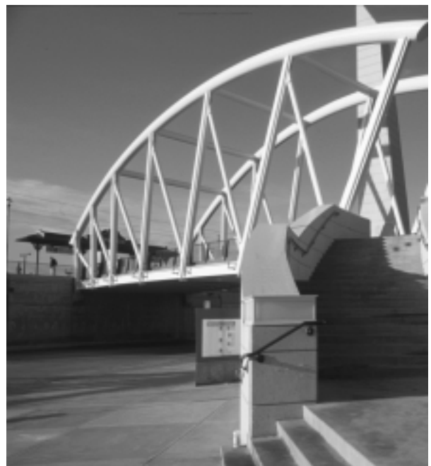
Englewood, Colorado, pedestrian bridge - part of Denver's regional transit system
